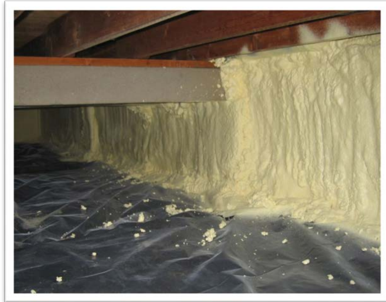
Conditioned crawlspace with air sealed and insulated walls
