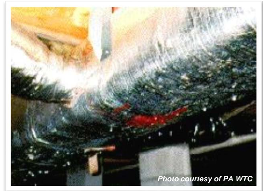
Water droplets of condensation on AC ducts
